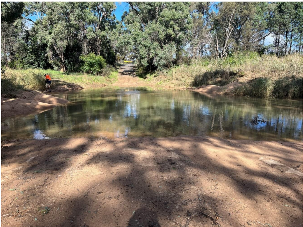
Photo 6 – Merrygoen Creek Causeway on Yarrow Road, Mendooran – 1 June 2022
