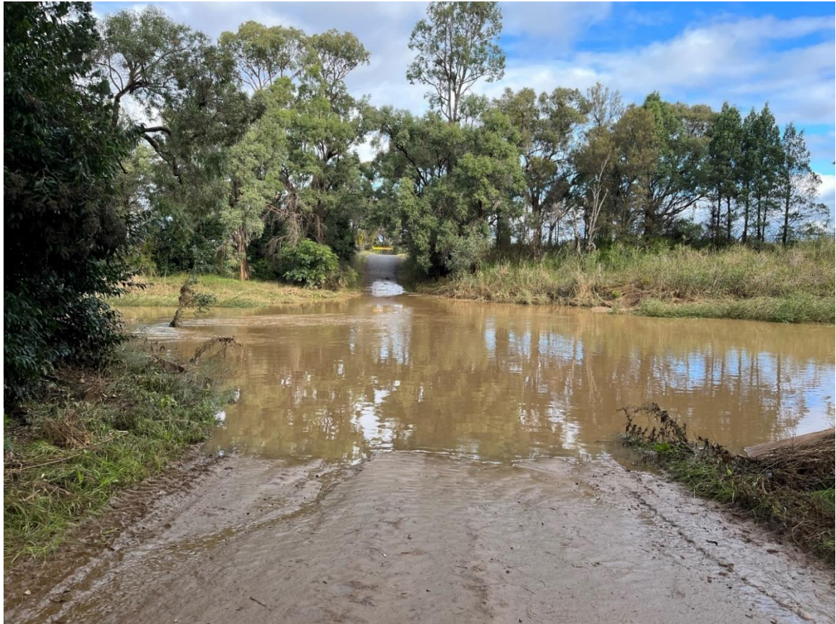
Photo 5 – Merrygoen Creek Causeway on Yarrow Road, Mendooran – 13 May 2022
