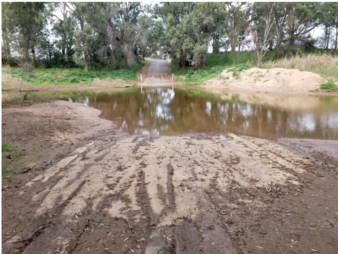
Photo 2 – Merrygoen Creek Causeway on Yarrow Road, Mendooran – 10 September 2020
