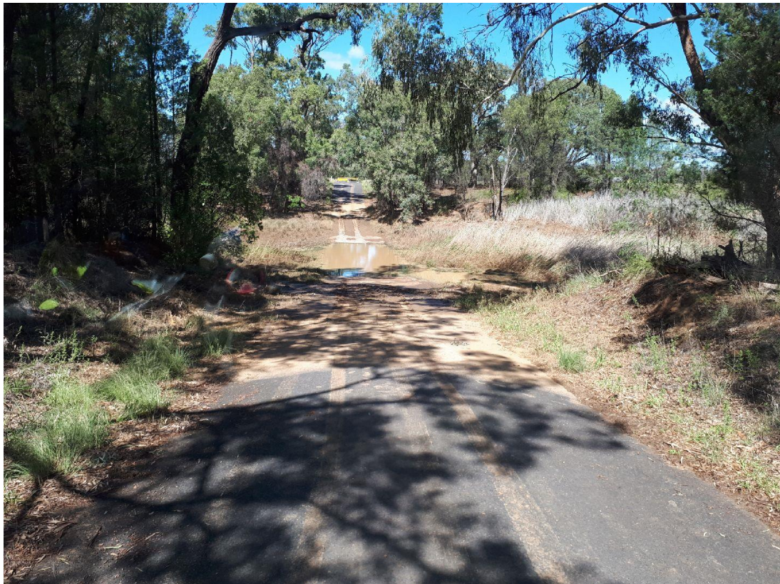
Photo 1 – Merrygoen Creek Causeway on Yarrow Road, Mendooran – 19 April 2019
