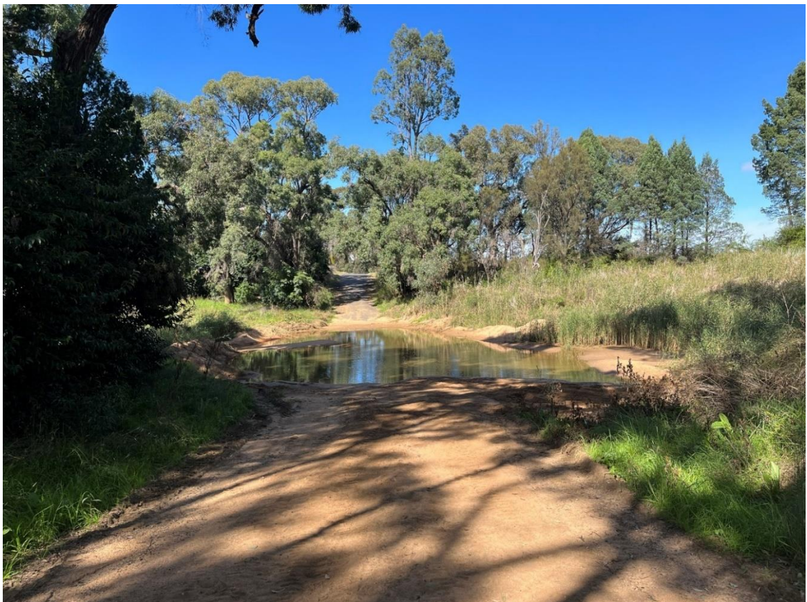
Photo 4 – Merrygoen Creek Causeway on Yarrow Road, Mendooran – 10 May 2022
